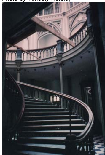
Rotunda Before Restoration Photo by Eean McNaughton
