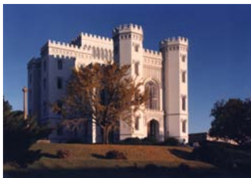
Exterior from Levee Photo by David King Gleason
